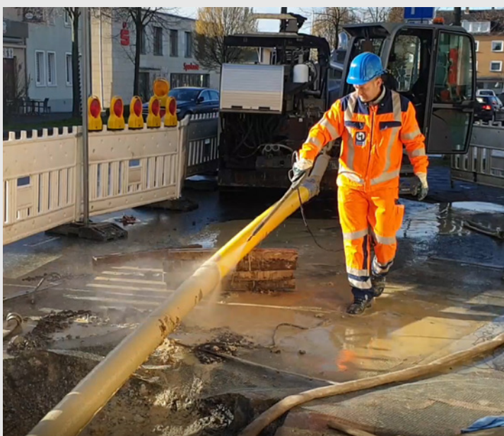
Figure 1: PA-U12 pipe OD 160 after installation by HDD in Beckum (Westnetz, 2019)
